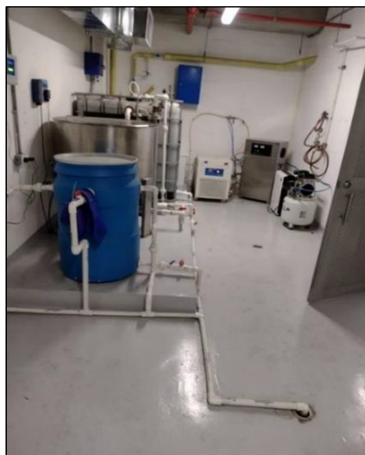
Figure 17. Photograph of the ozonation process installed at Imbanaco Medical Center
