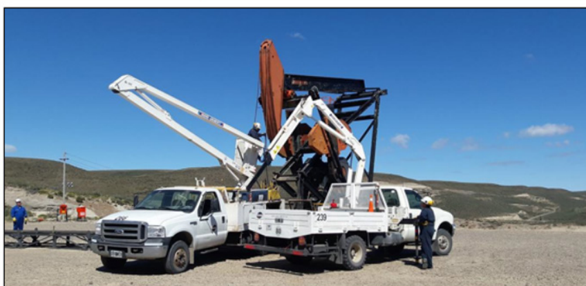
Figure 10. Two crews working together to change the strobe on the mule head
