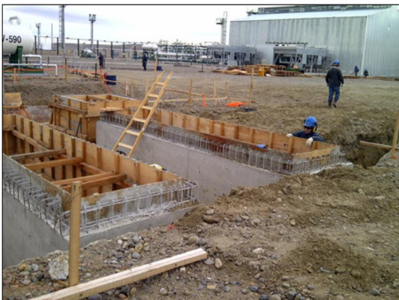
Figure 9. Chamber formwork
