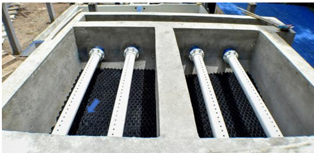
Figure 10. Laminar Settler
