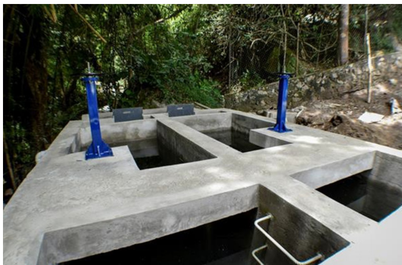
Figure 5. Sand trap structure
