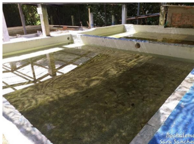
Figure 11. Upflow Fast Filter
