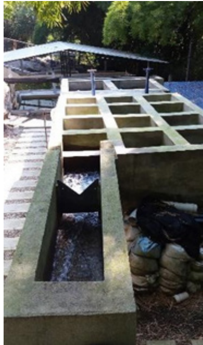
Figure 8. Parshall flume and Alabama type flocculator
