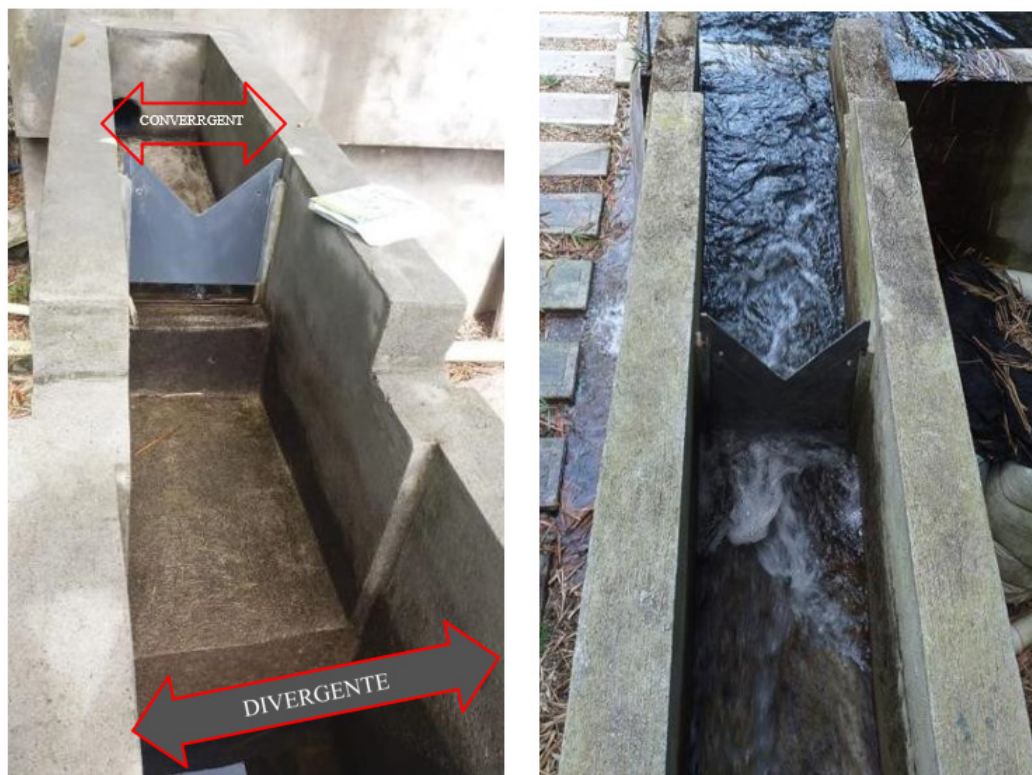
Figure 6. Inlet pipe and Parshall flume
